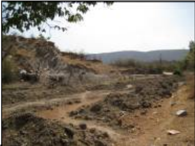
Once the mining is complete the new flattened land will be used as an agricultural field.
